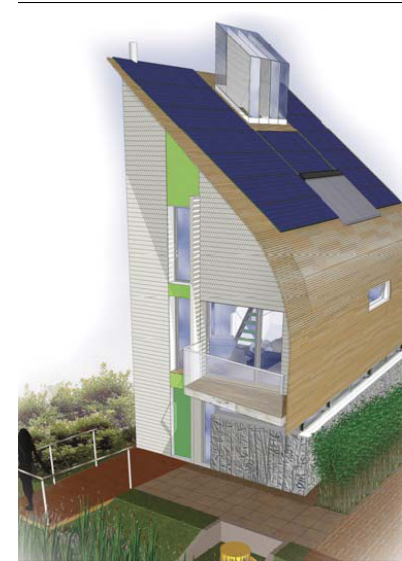
1.13 The simple barnlike form, derived from a 40 degree roof pitch accommodating a Photovoltaic (PV) array, which generates all the electricity for the house. The sweeping roof envelops the central space.
