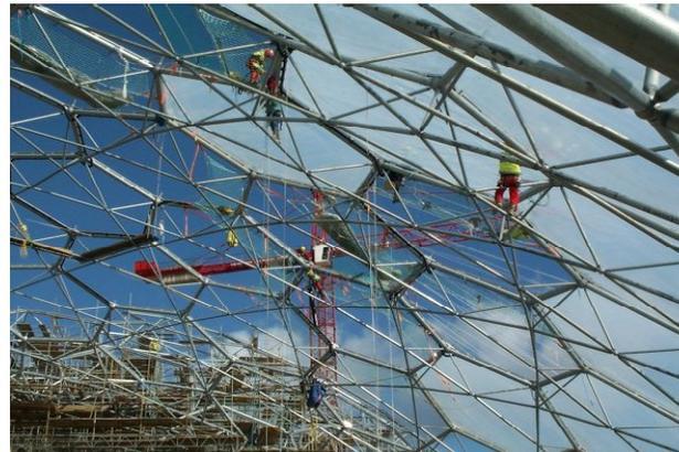
1.08 Installation of the ETFE pillows.
