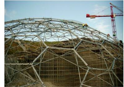
1.12 Construction of the steel hexagonal bracing
