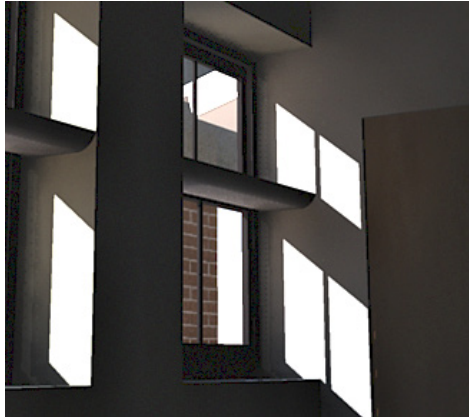
This image shows the lightshelves that were installed as part of our redesign.
