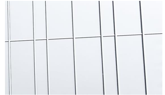
Actual material photo from COE building
