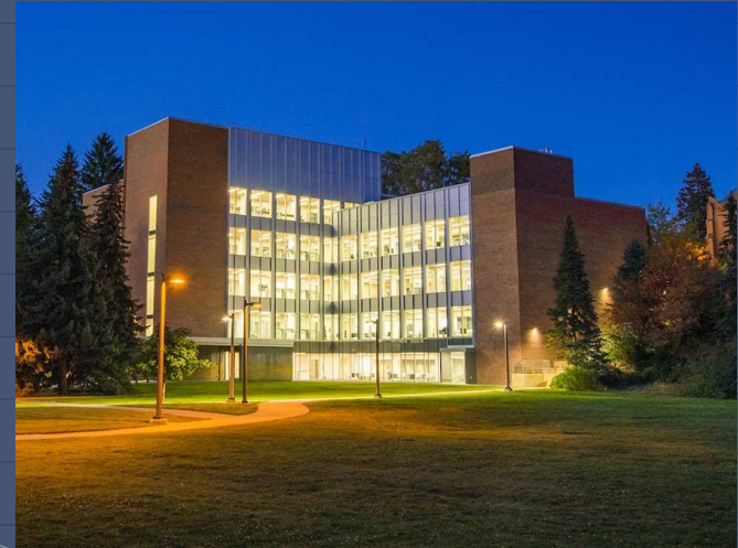
Education Building in 2016 ( After renovation) Source : https://www.uidaho.edu/ed
