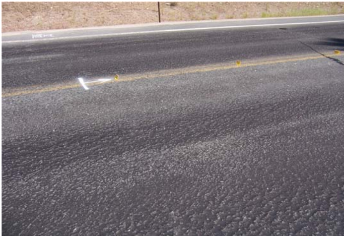
Condition prior to application
