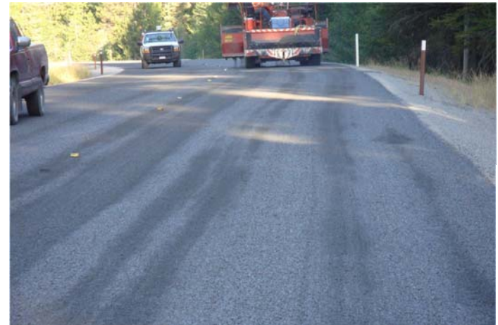
Second Seal – Day of placement (moist choke stone)
