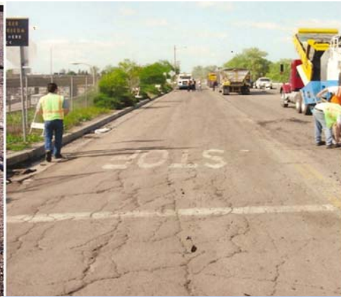
May 2003 During Installation
