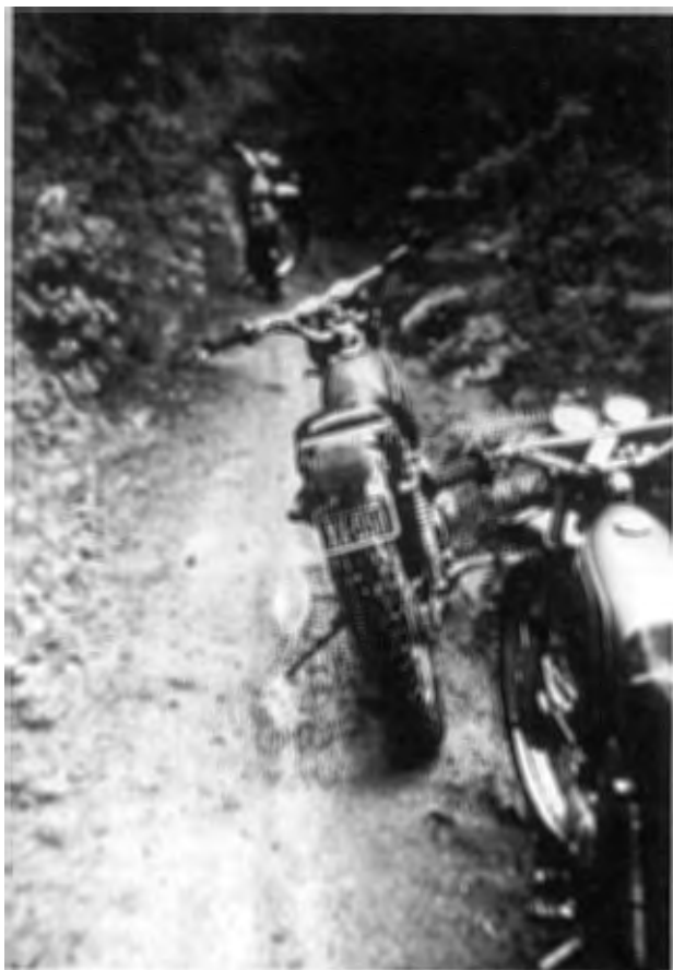
FIGURE 8. This motorcycle trail has been hardened in an inconspicuous manner with soil cement. (Photo: R. F. Washburne.)
