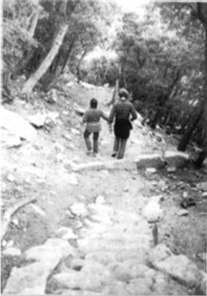
FIGURE 6. Rock water bars divert water off this trail in Yosemite National Park. The rock steps in the foreground also reduce the potential for erosion. (Photo: D. N. Cole.)
