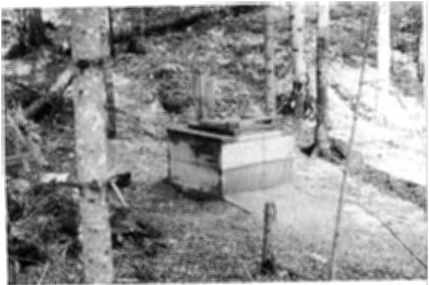
FIGURE 2. Pit toilets, if located on shallow soils and near water, can be a source of coliform bacteria and associated pathogens. (Photo: W. E. Hammitt.)
