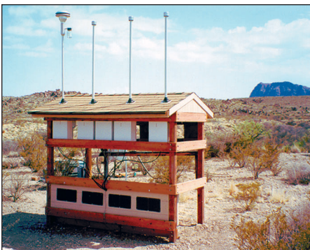
Aerosol samplers at Big Bend National Park, Texas. The chemical analysis of sample filters allows scientists to determine the contribution of various chemical species to visibility reduction in parks.
