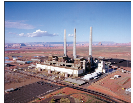
The Navajo Generating Station, located in Page, AZ, near Grand Canyon National Park, installed scrubbers in 1999 to reduce annual sulfur dioxide emissions by more than 60,000 tons. These reductions will result in better visibility at the Grand Canyon.
