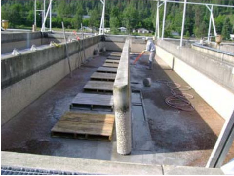
Removing center wall
