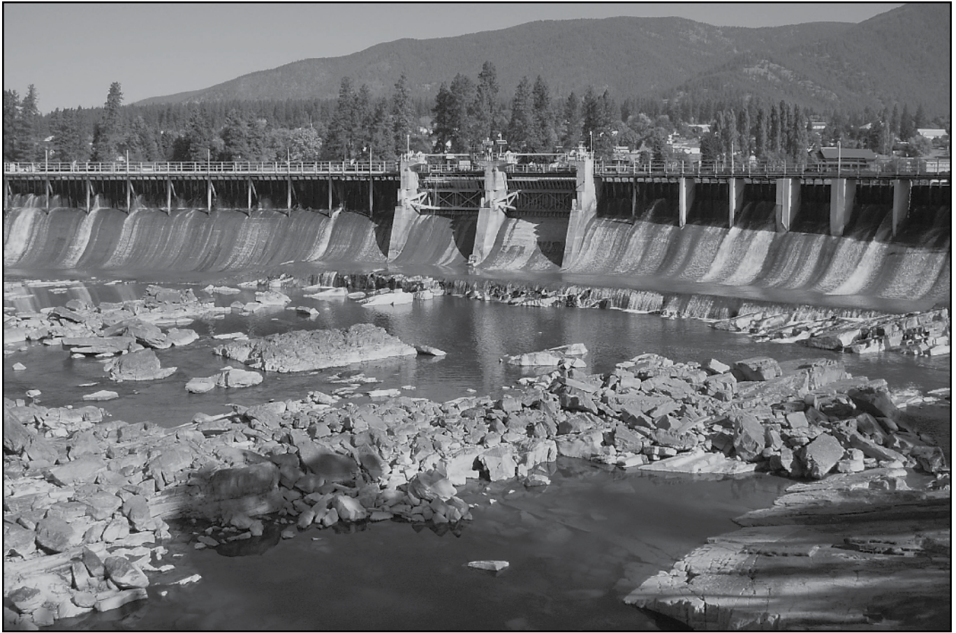
Low flow conditions at Thompson Falls Dam on the Clark Fork River, Montana, where no fish passage facilities are currently available.
