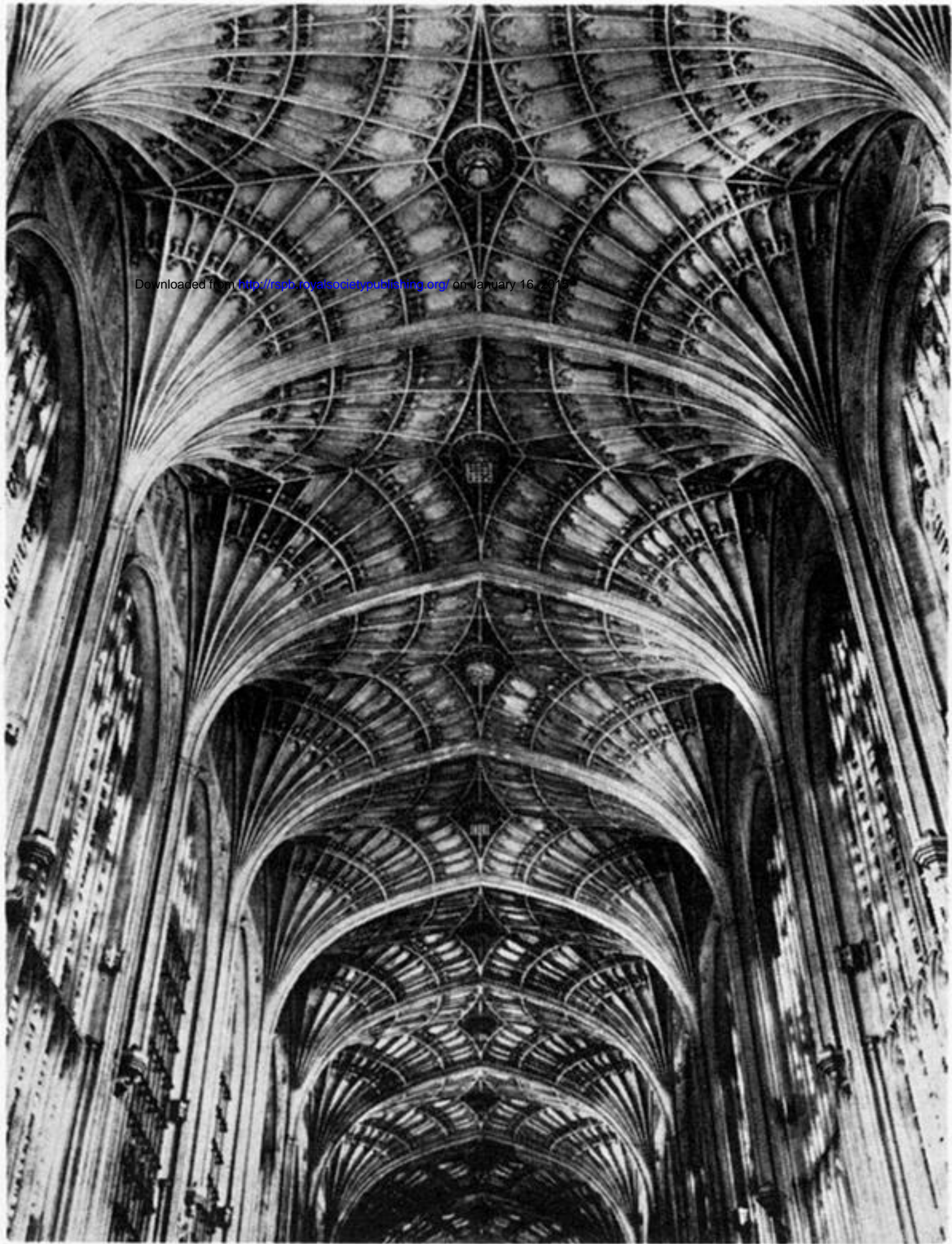
FIGURE 2. The ceiling of King's College Chapel.
