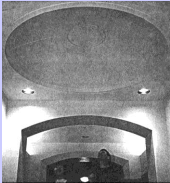
Dome over elevator lobby at UTexas produces surprising sound levels.
