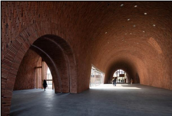
Traditional smoke holes used in ancient kiln design are adapted to bring in natural light or to hide artificial light sources.
