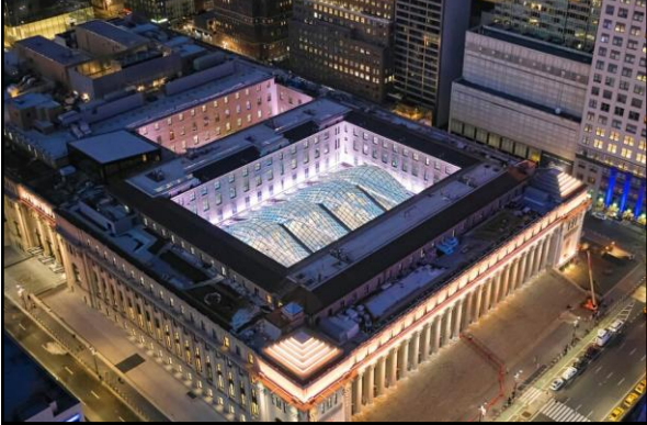
Daniel Patrick Moynihan Train Hall Honor Award • Interior Lighting • Design Team: Domingo Gonzalez Associates; SOM
