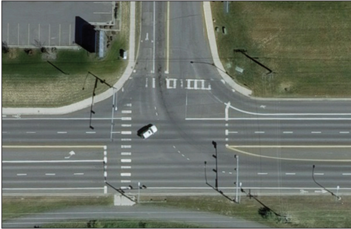
Figure 12. Aerial view of SH 8 and Warbonnet Drive
