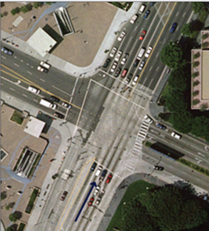
Figure 46. Aerial view of Lankershim Blvd. intersection
