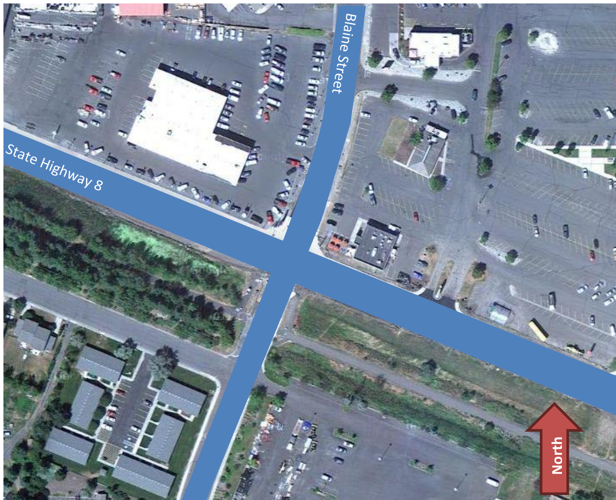
Figure 3: Intersection of State Highway 8 and Blaine Street in Moscow, Idaho
