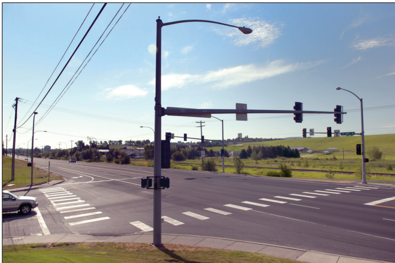
Figure 14. Mast arm, lighting, signs, and signal displays
