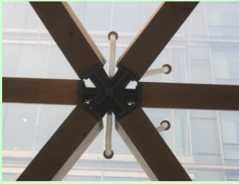
ETFE Glazing at Canary Wharf Crossrail Station
