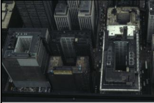
Light wells and crenellation
