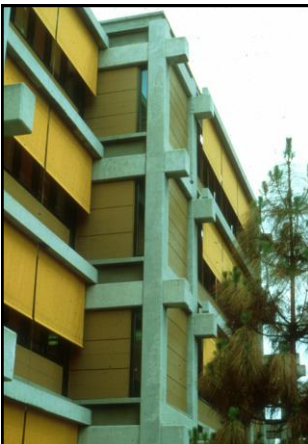
North windows use vertical fins (structure).
