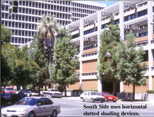
Case Study Bateson Building, Sacramento
