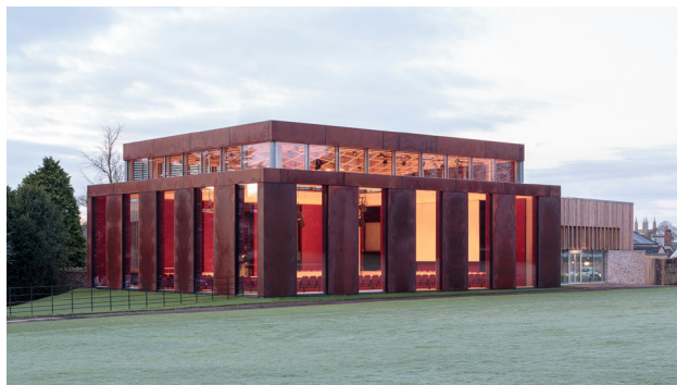
The recital hall's east and north façades.
