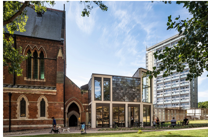
St. Mary Magdalene's addition has four bays of full-height double doors in its east-facing wall.
