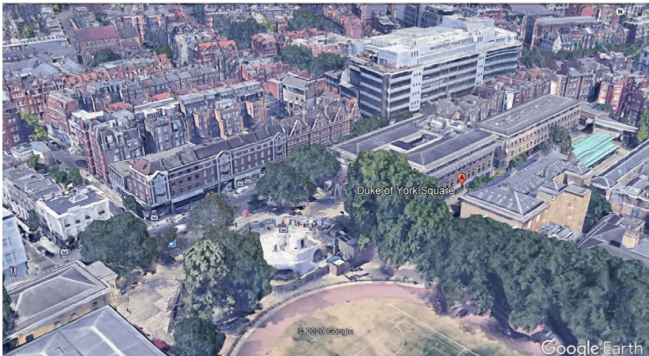
Here's the Duke of York Café under construction in its context in London.
