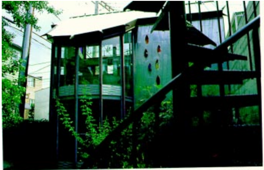
The glazing on the north side of the building affords a view to the garden, provides daylighting to office and library/conference areas, and the vent panels below the fixed glass of the bay allow cross ventilation.
