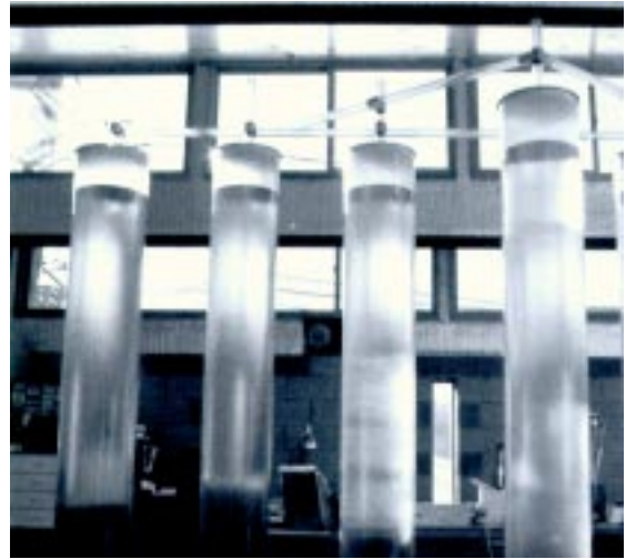
Water tubes used as thermal mass separate the principal's office from the drafting room.
