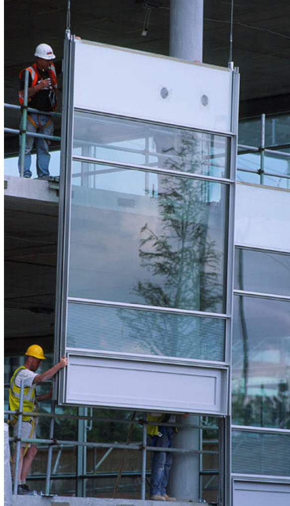
The module's panels from top to bottom: Opaque insulated, daylight, view, modesty, and opaque insulated.
