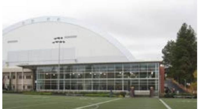
The Kibbie Dome addition has four bays of twenty-four panes of glazing in its east-facing curtain wall.
