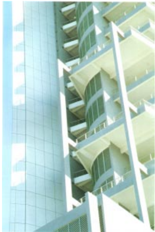
Air handling unit plant rooms viewed from the north.
