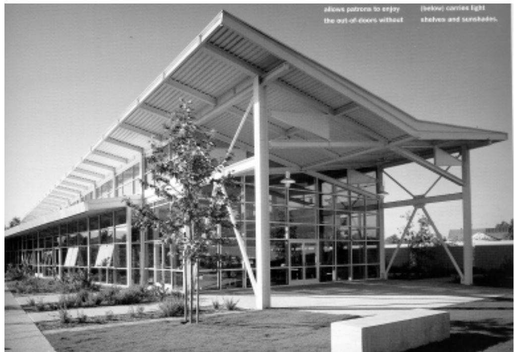
View of southeast corner of library from the garden courtyard.
