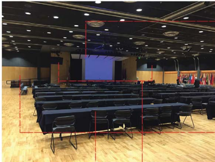
01 Gypsum board Overing hanging above the stage to reflect sound
