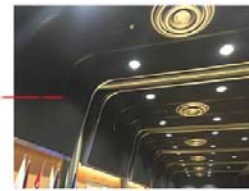
01 Absorbing Ceiling Panels The absorbing ceiling panel are covered entire space in order to reduce the sound reflection
