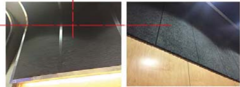
02 Acoustic Panels Two types of acoustic panels cover upper of the surrounding walls
