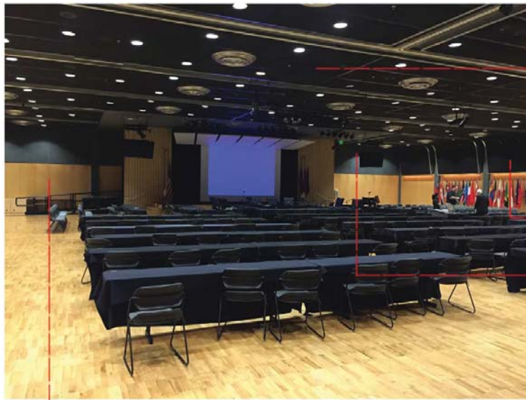
01 Absorbing Ceiling Panels The absorbing ceiling panel are covered entire space in order to reduce the sound reflection
