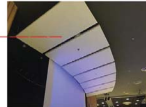
01 Gypsum board Overing hanging above the stage to reflect sound
