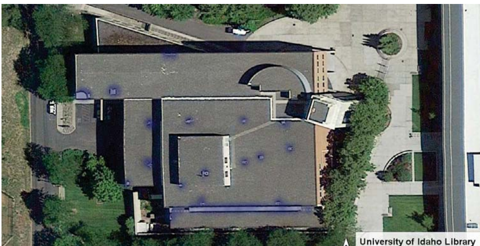
Highlighted Drainage Collection Units Located on top of the Roof Structure
