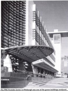
The PNC Financial Center in Pittsburgh was one of the green buildings analyzed.
