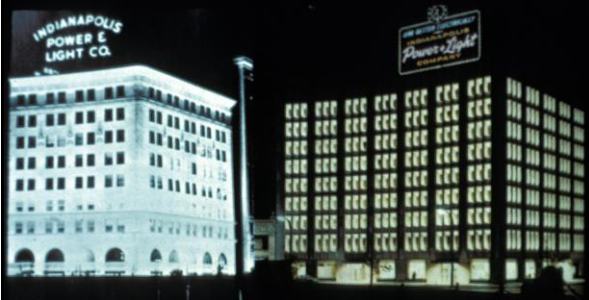
...before and after 1960s remodel...
