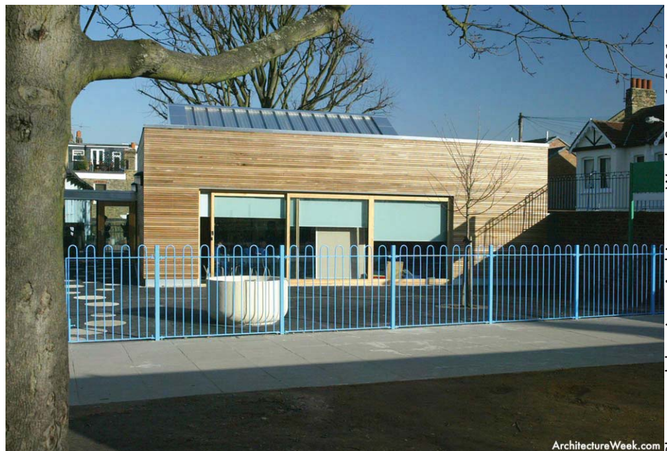
Both the south-facing aperture and the roof of the north-facing clerestory can be seen from the street.
