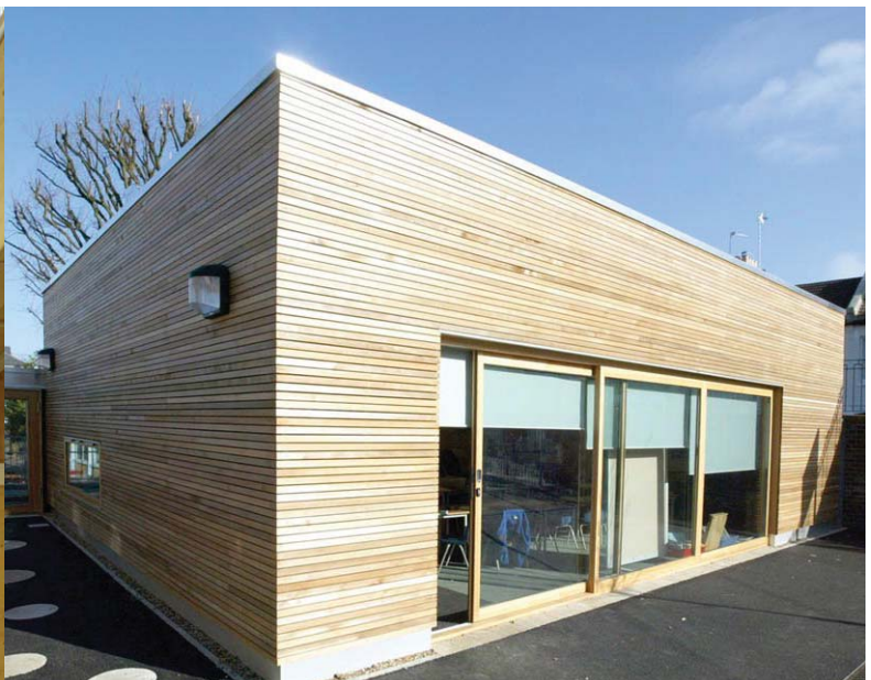
View of classroom's southwest corner.
