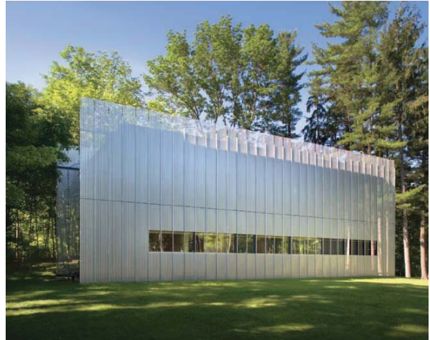
The perforated screen on the south facade seems solid in the daylight.
