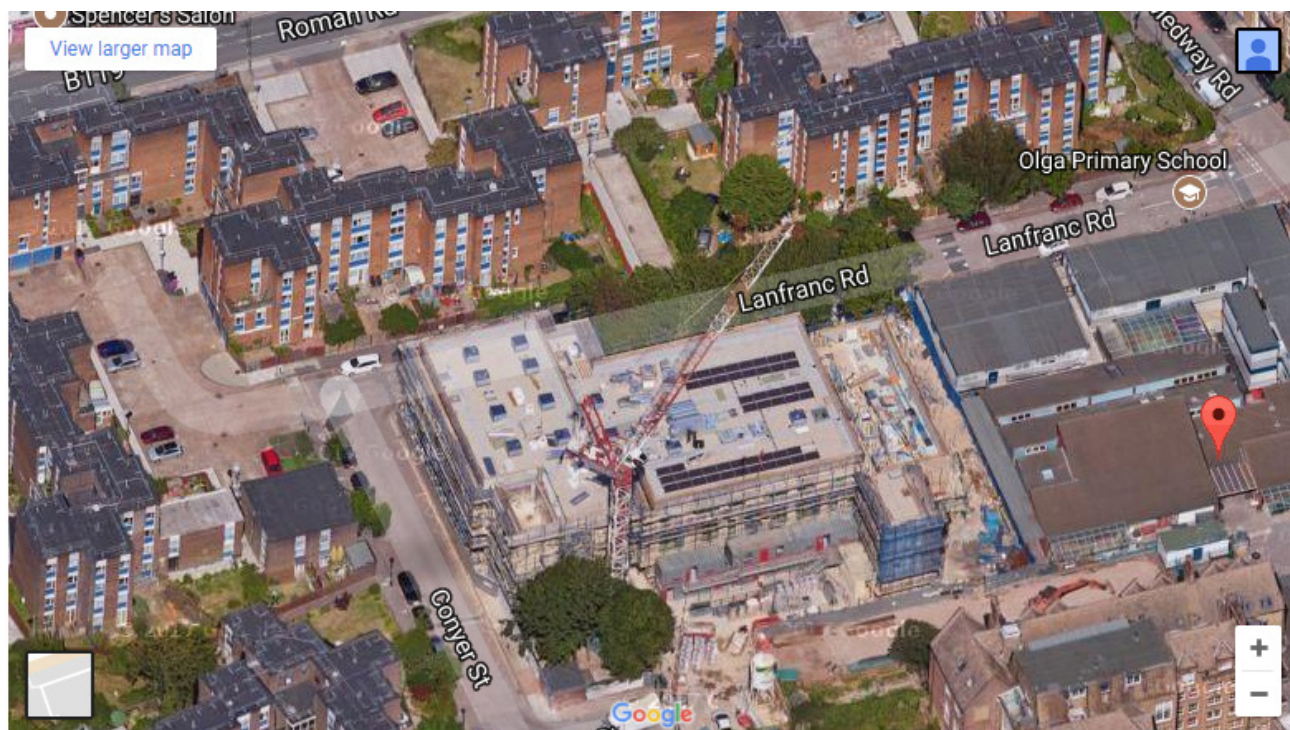
Olga under construction, north is up.
