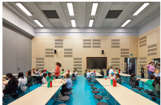
The large hall is used as a cafeteria. The black rectangles in the ceiling are two of the four skylights (black out mode). The movable wall to the left separates it from the small hall.
