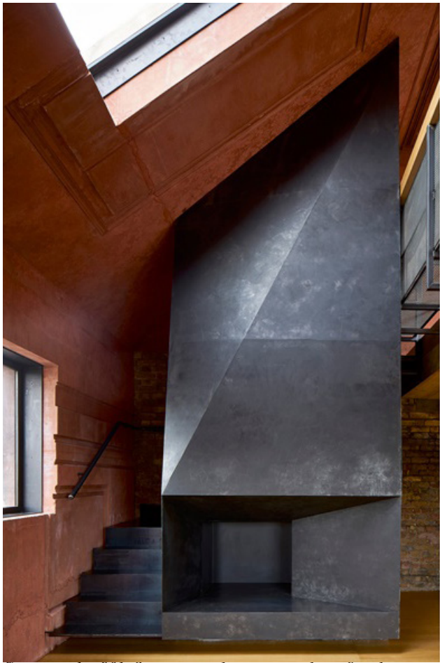
Stairs to the fifth floor wrap the cast-in-place fireplace. An east-facing roof window lights the two-story void.
