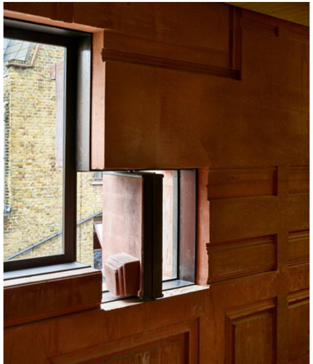
All of the windows but one are fixed-glass, but some like the one pictured are accompanied with pivoting operable vents.
