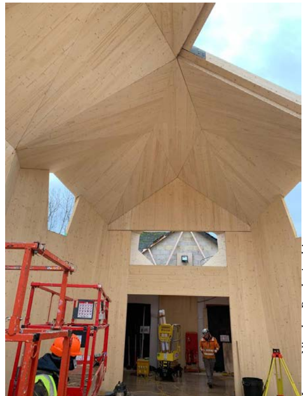
The CLT Stroud Chapel under construction.
