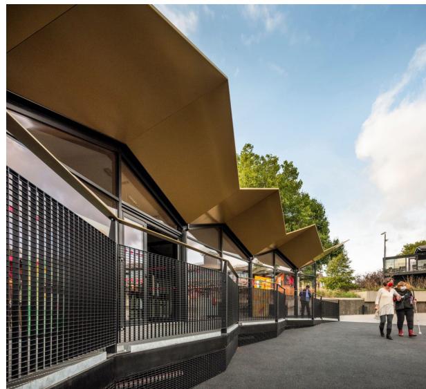
North facade of the NW2 pavilion.
