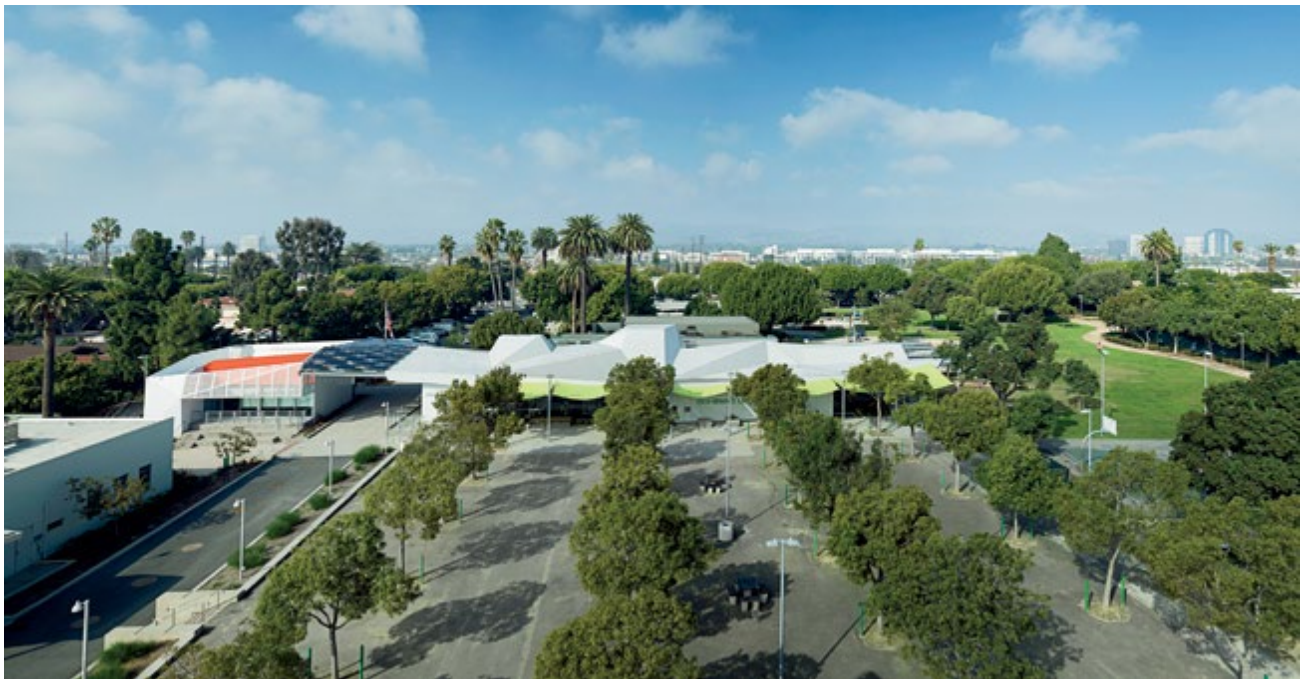
Looking Northwest, a PV-studded trellis connects the library to its freestanding community room.
