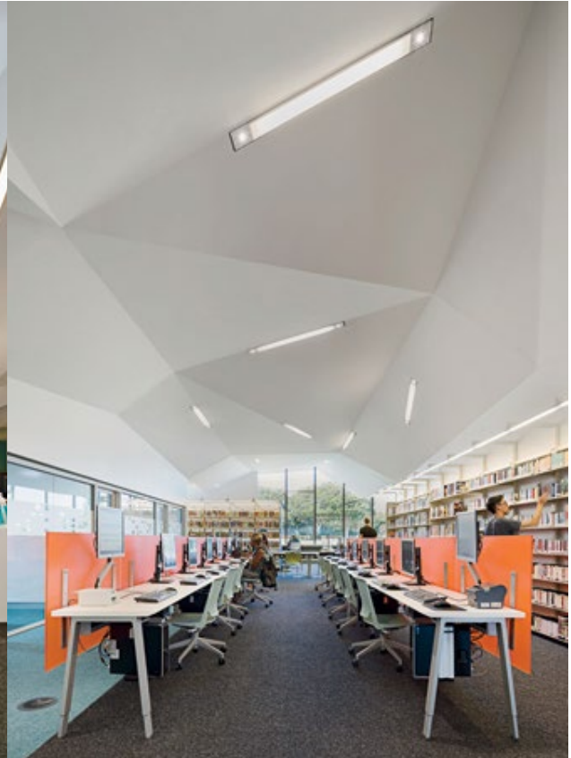
The reading room's faceted ceiling of noise-deflecting plaster is embedded with LED lighting.
