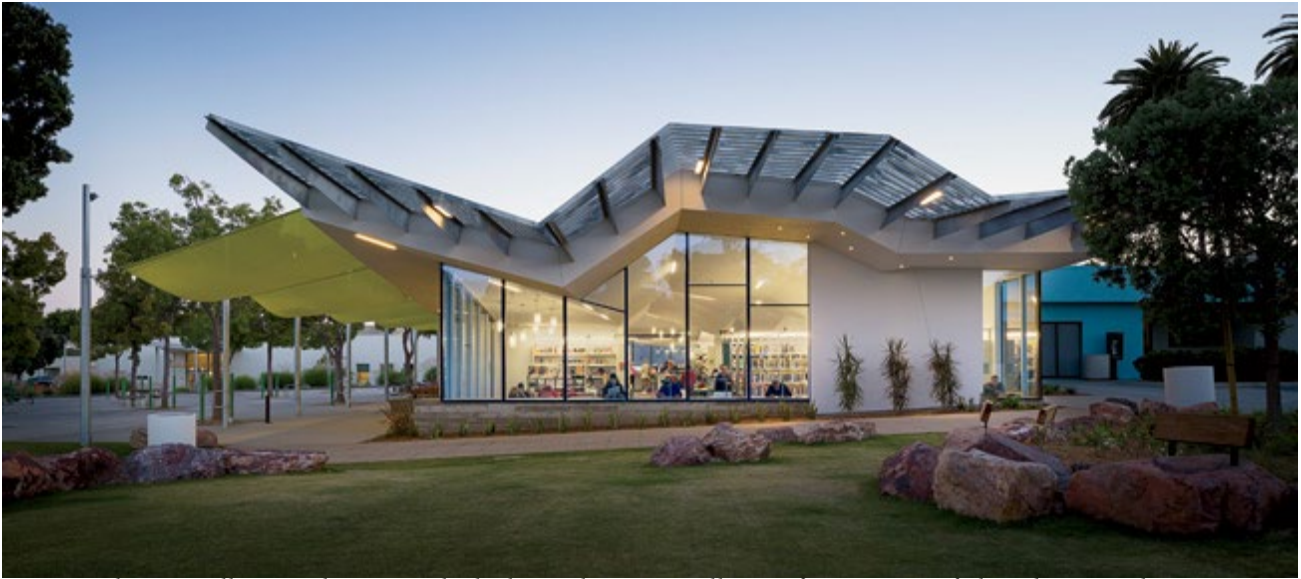
Deep overhangs, trellises, and awnings shade the reading room, allowing for expanses of glass that open the interior to daylight and immersive park views.
