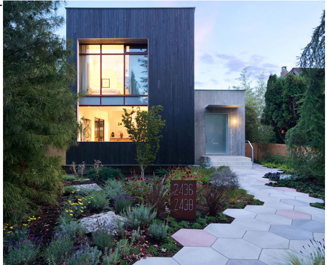
Front elevation (north facing) of Rough House showing its landscape design.
