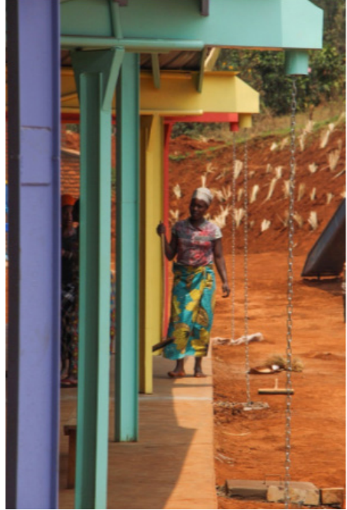
North edge of school with scuppers and rain chains fabricated using recycled material from dismantled Rwanda Trading Company factory at Rwandex.
