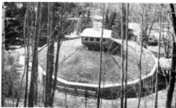
View of earthcovered roof looking south.
