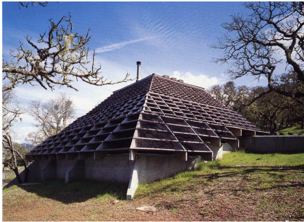
Obie Bowman nestled the pyramid into the sparsely forested landscape. He screened the exterior with redwood louvres and clad the southeast facade in air-based solar panels. A central hearth supplies heat when solar gains are not adequate for solar heating.
