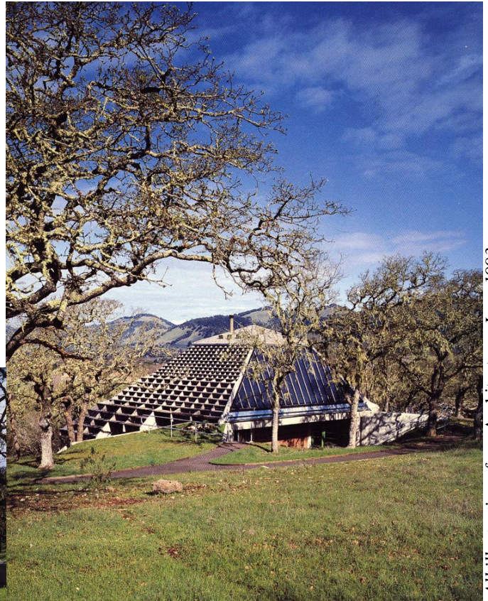
Obie Bowman nestled the pyramid into the sparsely forested landscape. He screened the exterior with redwood louvres and clad the southeast facade in air-based solar panels. A central hearth supplies heat when solar gains are not adequate for solar heating.
