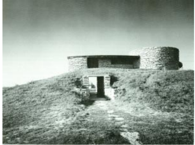
Entry tunnel viewed from north.
