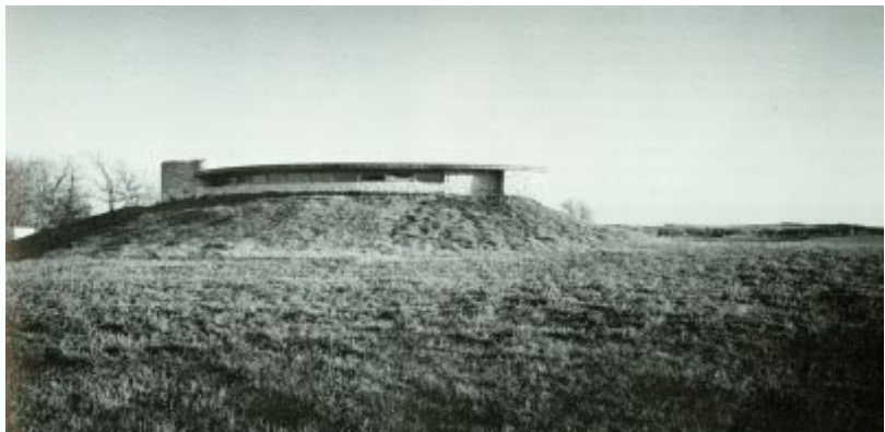
The northern berm rises almost to the level of the mezzanine windows. The sunken garden to the south, the concave shape of the house, and the slope of the roof and berm combined to produce high pressure pocket of still air that protects the house from winter's prevailing SW winds.
