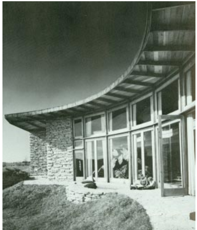
Curved south facade exposed to midday winter sun.
