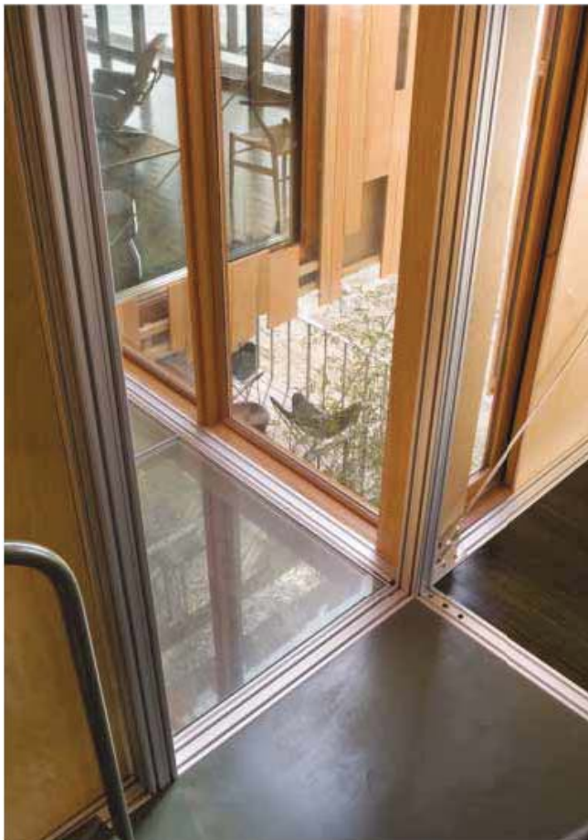
A clear glass bridge (right) connects the two halves of the house, spanning a garden landscaped with bamboo and gray stones.
