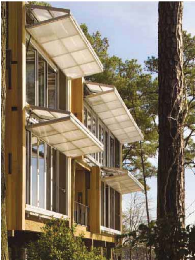
Operable hangar door shades on west facade (left), vertical cedar boards filter light on east (south & north too) facade (above), and all west window walls are fully operable (below).
