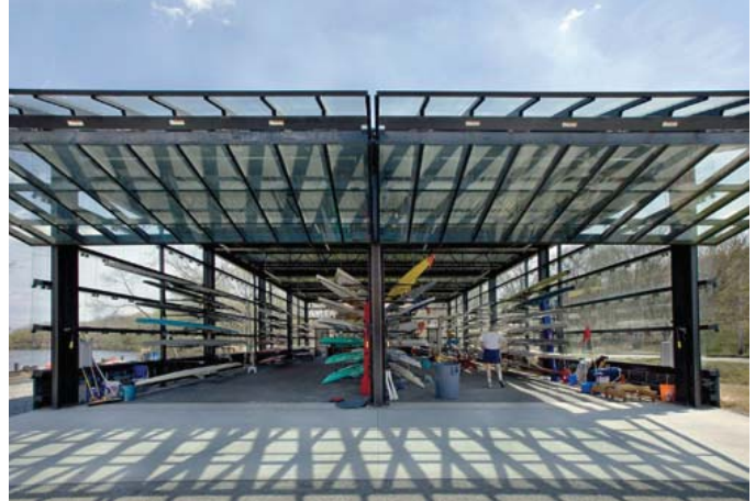
The glass-clad, steel-framed Ruth W. Somerville Sculling Pavilion houses the one- and two-person sculls and shells.
