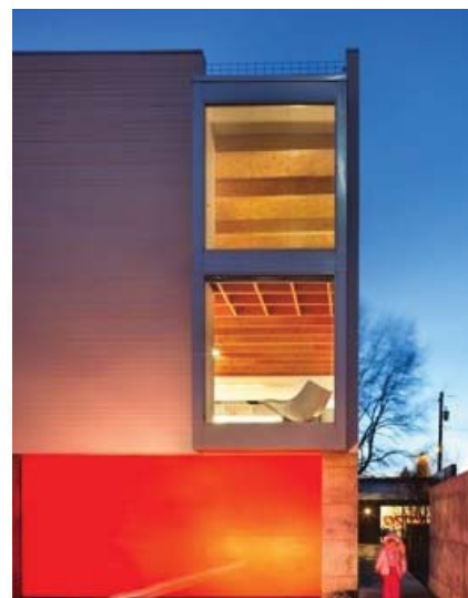
East facade and south side walkway.
