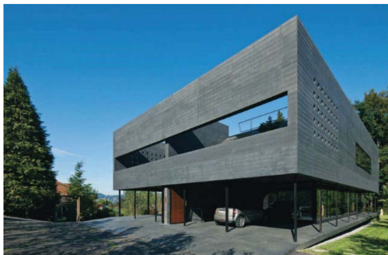
Southwest corner showing glazed enclosure of ground floor and concrete enclosure of second floor poised on slender steel pilotis.
